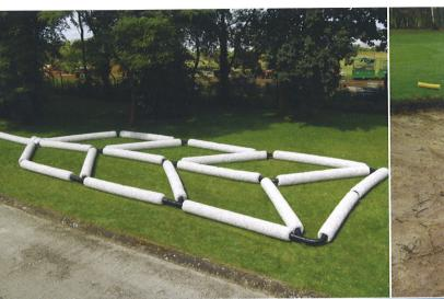
At the heart of the Polybed System is a geosynthetic aggregate, known as EPS aggregate, manufactured from recycled expanded polystyrene and engineered for optimum performance with consistent form.
